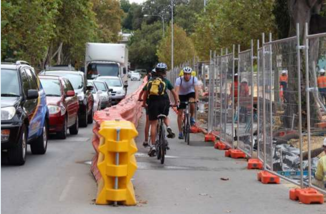
Figure 4: Temporary shared path provided during the Elizabeth Quay construction
