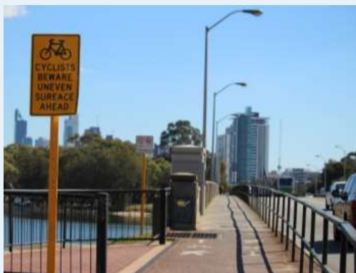
Figure 2: A section of the Causeway shared path is narrow and does not meet Austroads guidelines of a minimum shared path width of three metres
