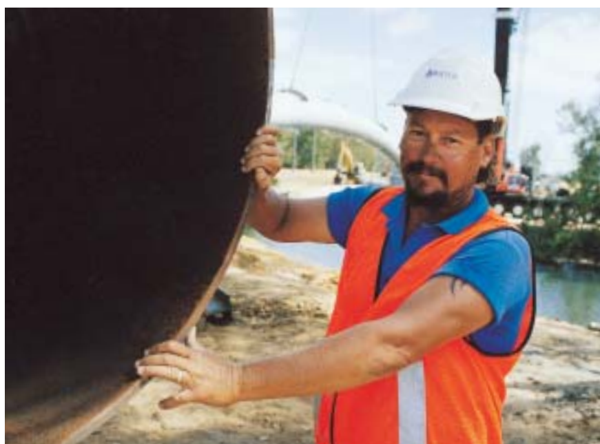
Laying pipe along the 106km Stirling Trunk Main
