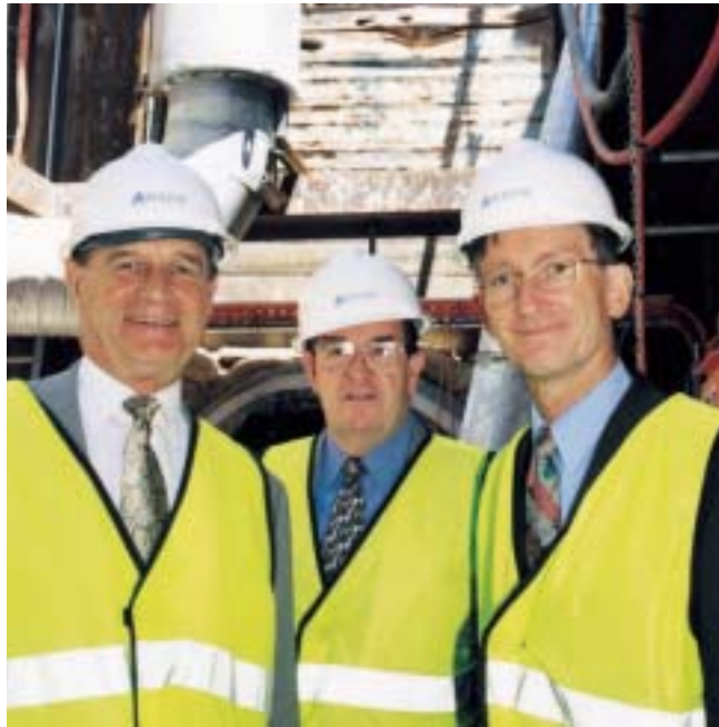
Lt-Gen. John Sanderson, Governor of Western Australia, with Water Corporation Chairman Peter Jones and Managing Director Jim Gill, inspecting work on the Perth Main Sewer
