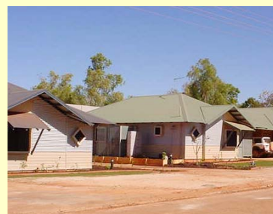
Teachers' housing ... some of the six new 2-bedroom GEHA dwellings built in Fitzroy Crossing to ease the accommodation shortage.
