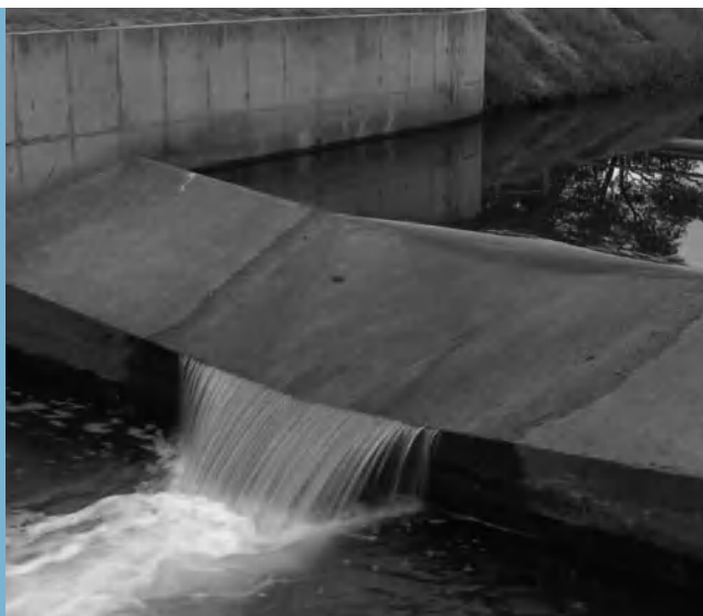
Gauging stations, maximum height recorders and rain gauges monitor continuous flow, peak flow and rainfall data retrospectively, to calibrate our engineering models and assess requirements for flood protection.
