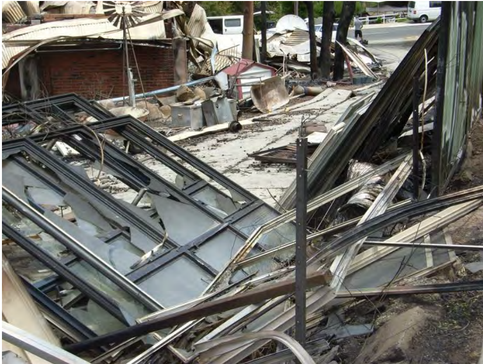
Photograph of burnt debris located on a private property 90
