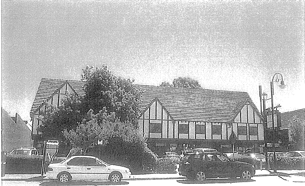
Tudor Building approx. 14 metres in height
