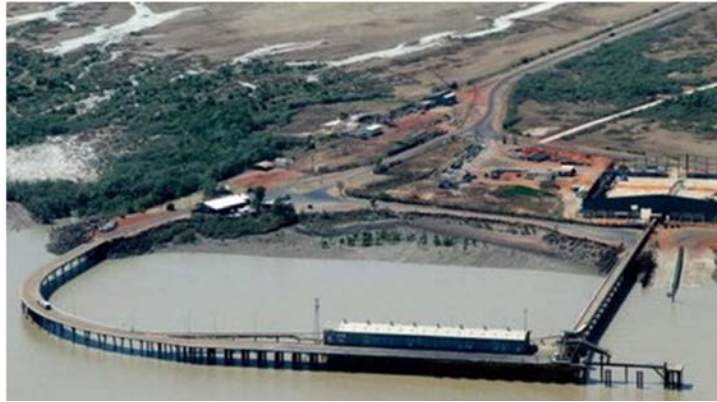
Figure 5 - Derby Wharf Infrastructure
