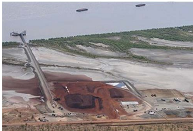
Figure 7 - Kimberley Metals Group Barge Loading Facility
