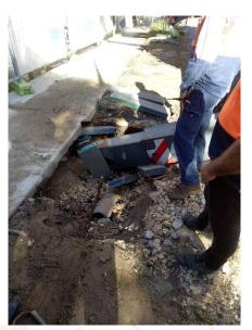
Following an incident on Monday 26/06/2017 where a slewing mobile crane tipped over due to an out rigger breaking through a water pipe the CFMEU recommend the following when setting up mobile cranes and truck mounted concrete placing booms:
