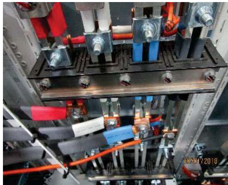
CUBIC's specially developed assembly bolt, it is not necessary to drill holes or cut threads. The assembly bolt allows for an adjustable connection, exactly where it is needed on the busbar holders. All busbar joints are designated as maintenance-free according to DIN 43671.
