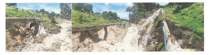
The gradient of the Scarp and the retaining sides of the landfill are so steep it seems impossible to be erosion free, with regular inundations to the Conservation Park, Banksia Rad and surrounding farms.
