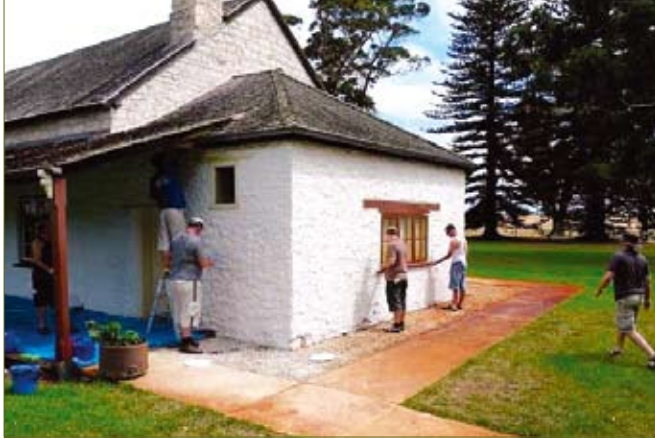
Volunteers from the WA Rover Scouts applying limewash to the laundry c.1925 at Wonnerup on the Labor Day long weekend Photo: G & M Dunn / National Trust
