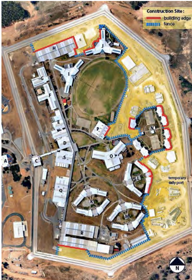
Figure 3: The internal construction site
