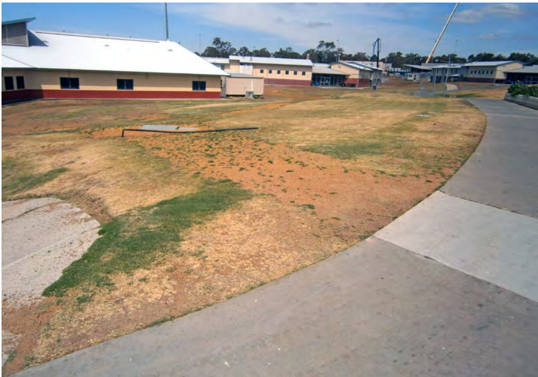
Figure 1: The poor state of the grassed area as a result of the expansion and the reticulation system not working.
