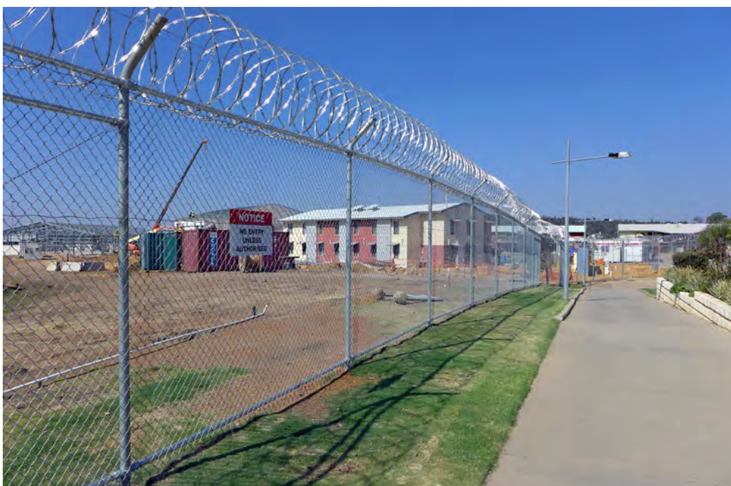
Figure 4: Internal demarcation fence separating the main prison from the construction site
